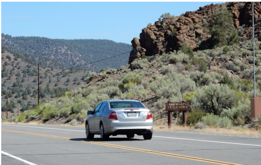
Near East Walker Stock Drive at PM 6.00
