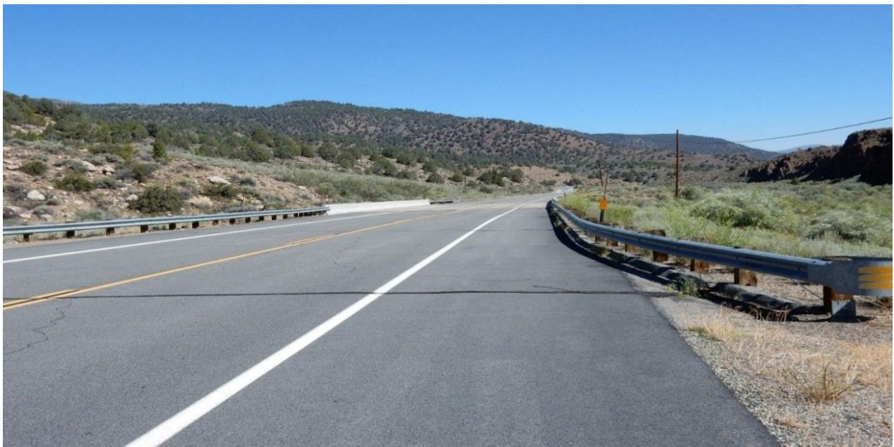
East Walker River Bridge at PM 6.20
