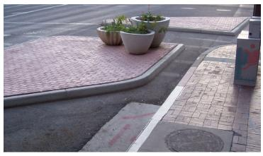
This curb extension allows water to drain to the sewer inlet, following the existing drainage line.
