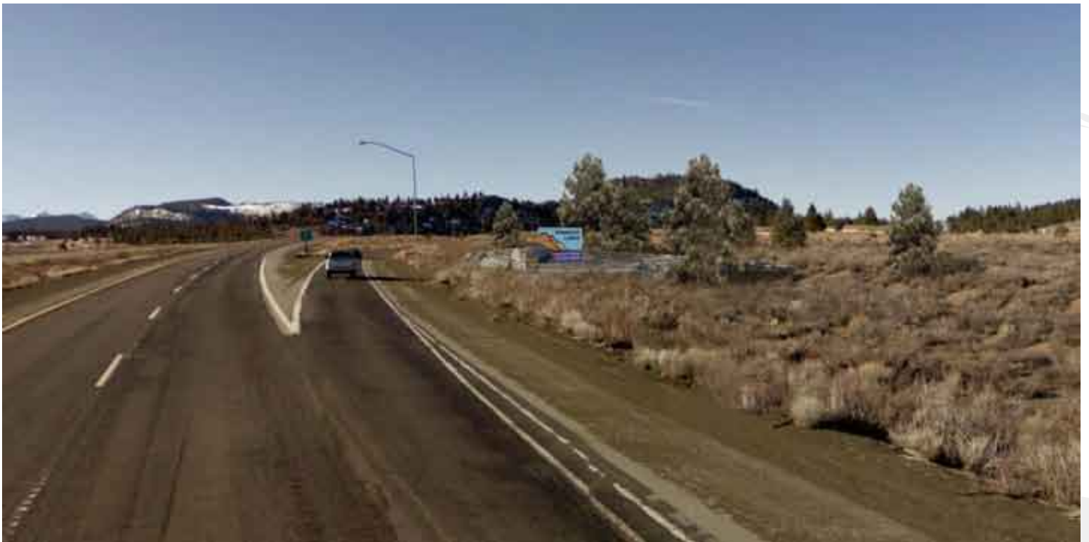
Mammoth Lakes Interchange After Enhancements
