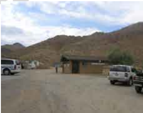
Public Restrooms at Park in Walker
