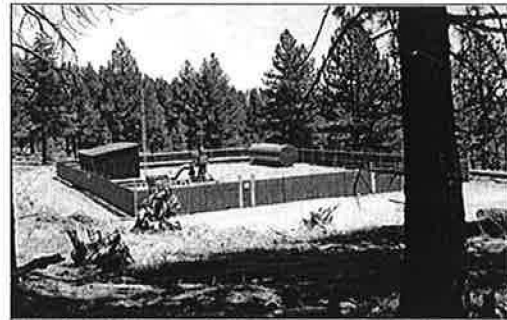
Photo of existing Geothermal well pad.
