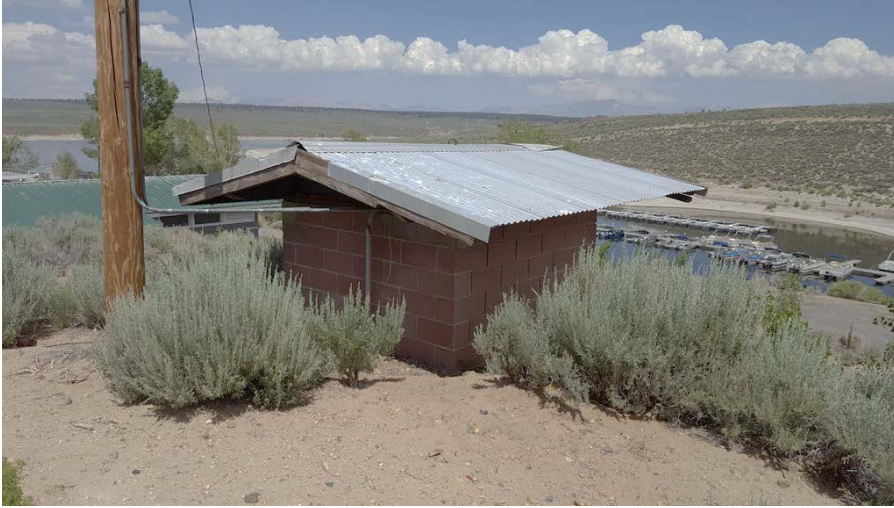
Figure 33. Well House, view toward northeast.
