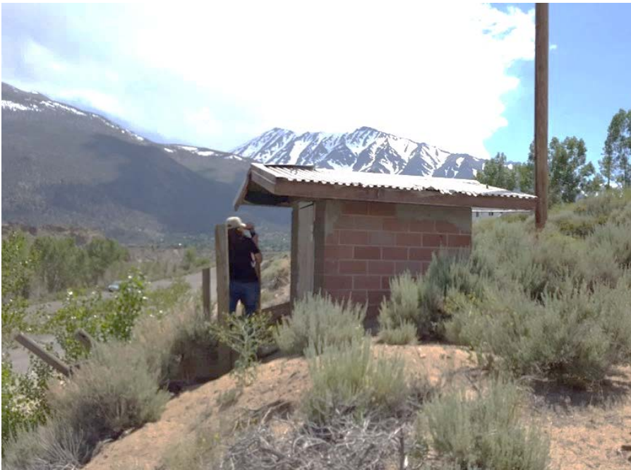
Figure 34. Well House, view toward south.
