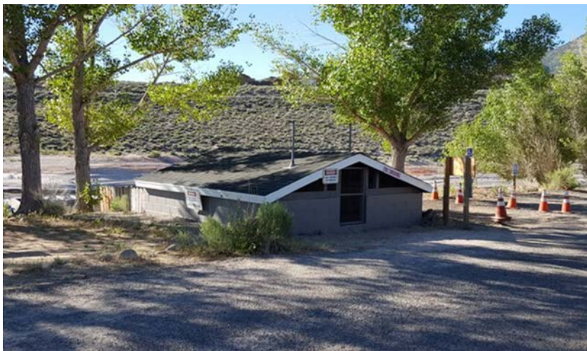
Figure 36. Fuel Facility, view toward southeast.
