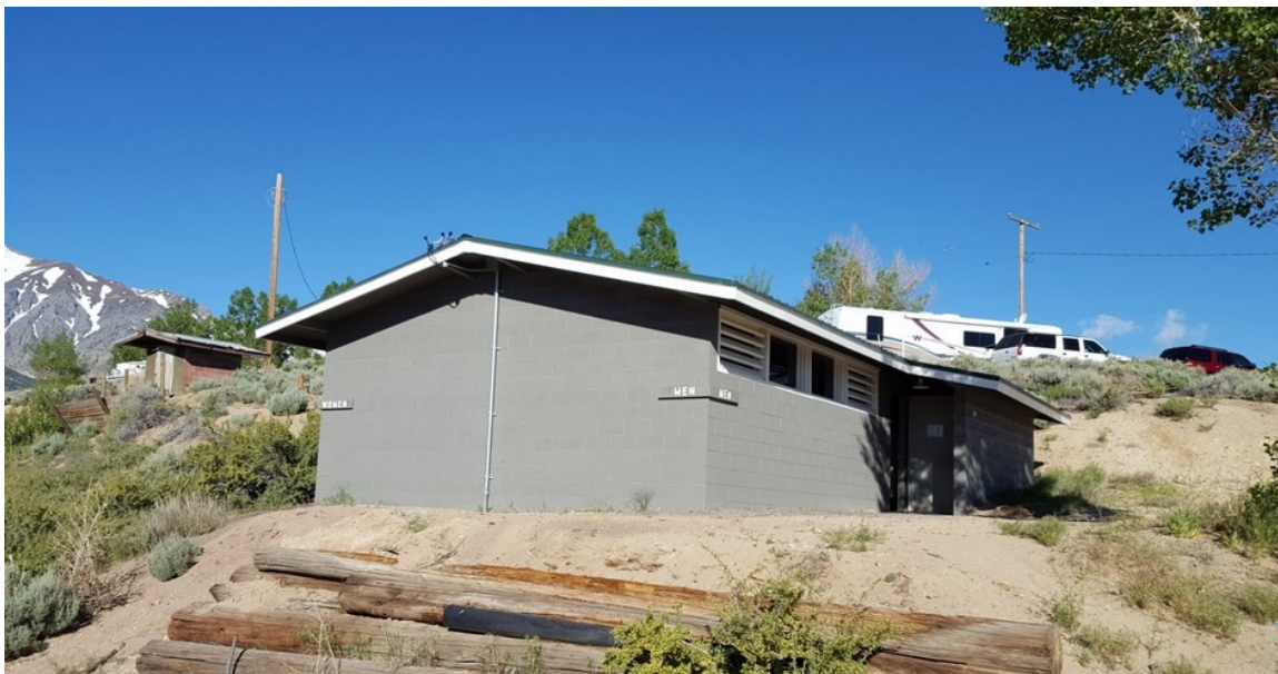
Figure 41. Public restroom, view toward southwest.
