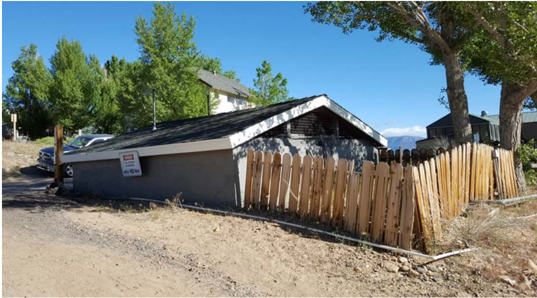
Figure 35. Fuel Facility, toward northwest.
