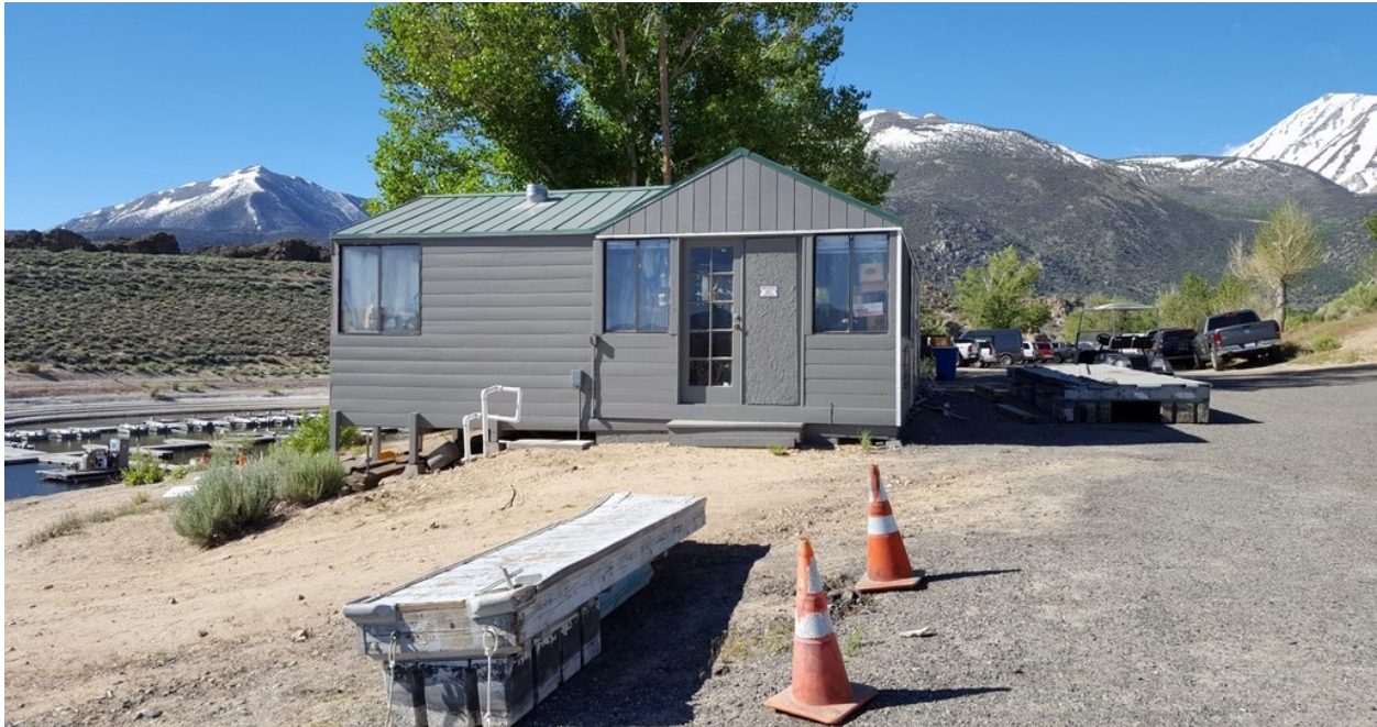
Figure 37. Boathouse/Storage Building, view toward south.
