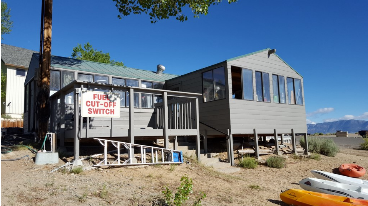
Figure 38. Boathouse/Storage Building, view toward northwest.
