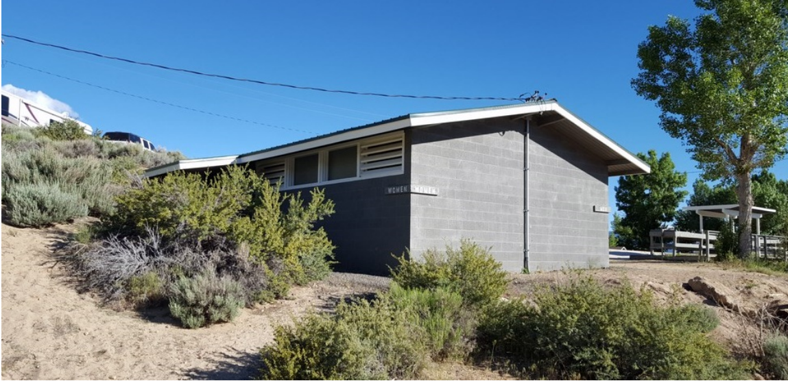
Figure 40. Public restroom, view toward northwest.
