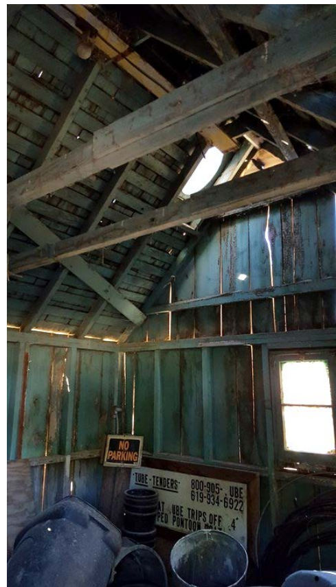
Figure 43, above. LADWP cabin/shed, view to southeast. Figure 44, below right. Interior of cabin, showing scabbed ceiling joist and one of two chimney-type openings in the roof.
