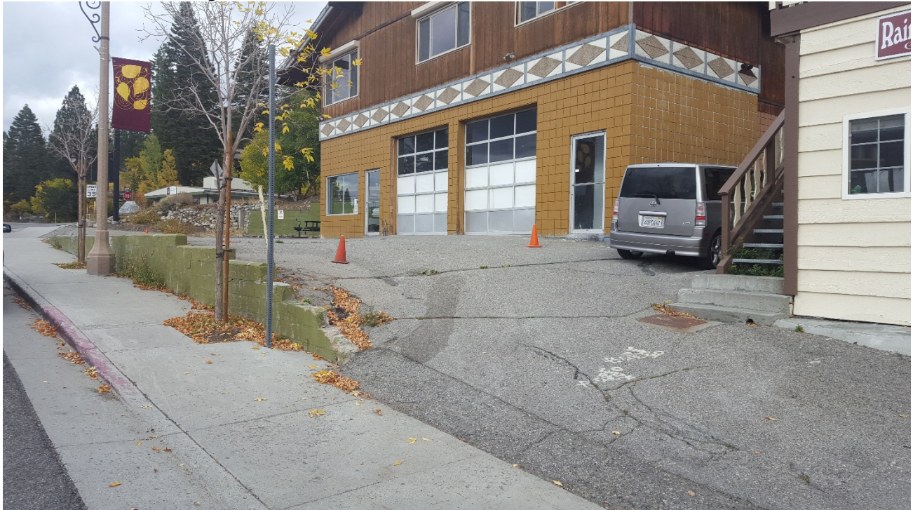
Photo 2: Front of building
