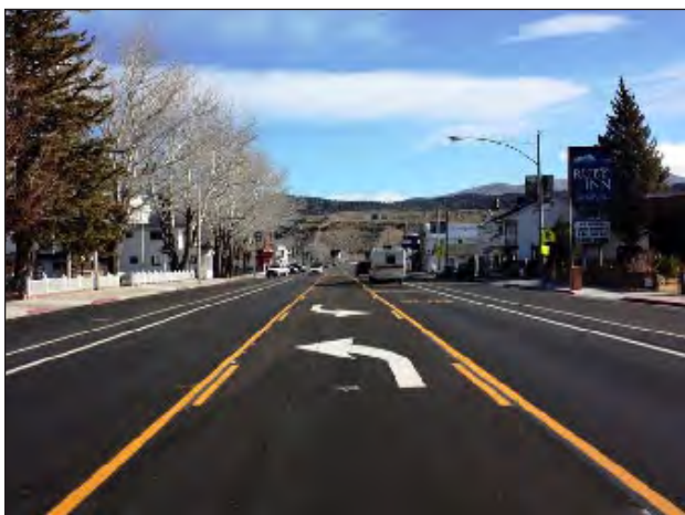
Looking west at the western entrance to Bridgeport just after repaving.
