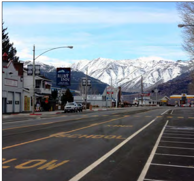
Bike lanes near reverse angle parking, where drivers leaving parking can see cyclists.
