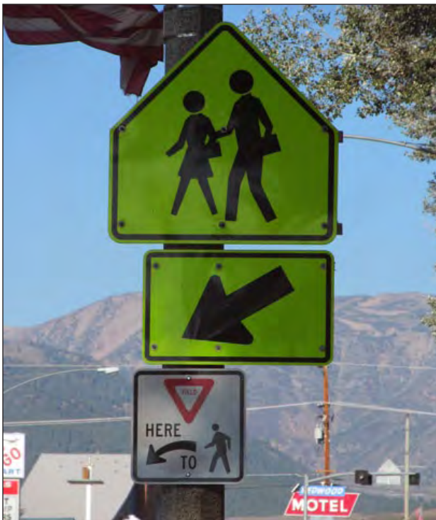
Pedestrian alert signs should better highlight the legal requirement that drivers MUST yield.
