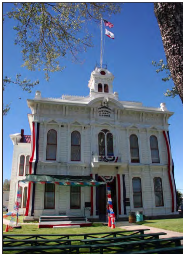
The Mono County Courthouse in 2012 dressed up for the July 4th parade.
