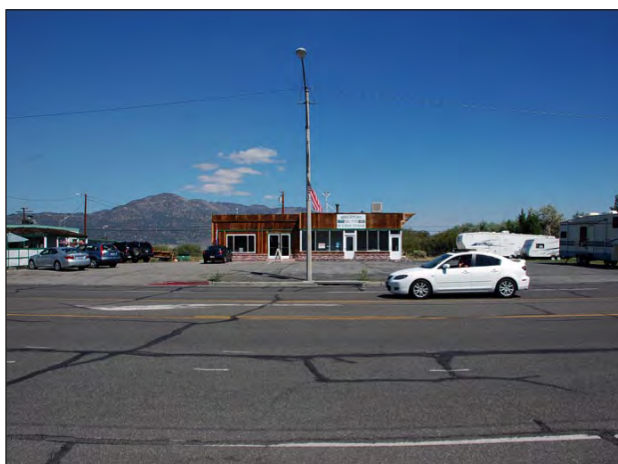
The one-acre boat storage facility on the eastern end of Main Street is a great opportunity.
