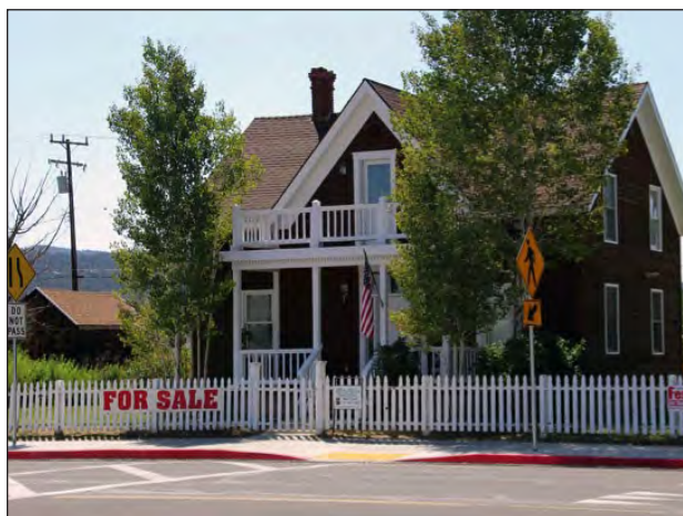
The front of a large property on the eastern end of Main Street.
