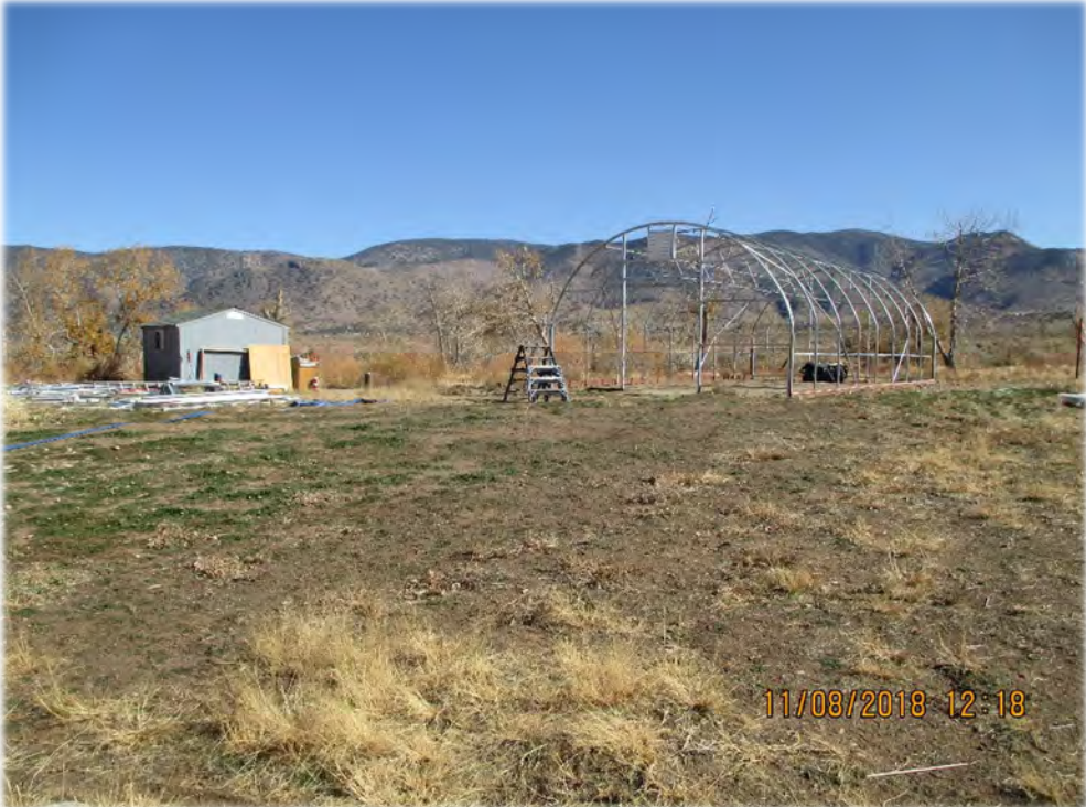
Photo 2. Looking to the southeast. The metal frame structure is one of the proposed immature plant areas. The wellheads are located directly adjacent to the gray building.
