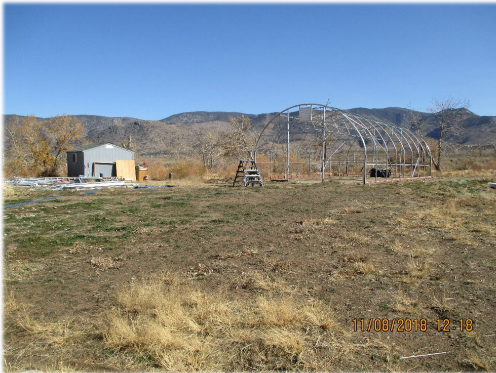
Figure 4: Looking to the southeast. The metal frame structure is one of the proposed immature plant areas. The wellheads are located directly adjacent to the gray building.
