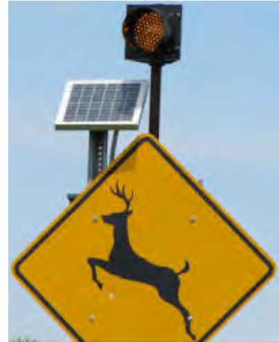
Image 9: Standard deer warning sign with flashing beacon.
