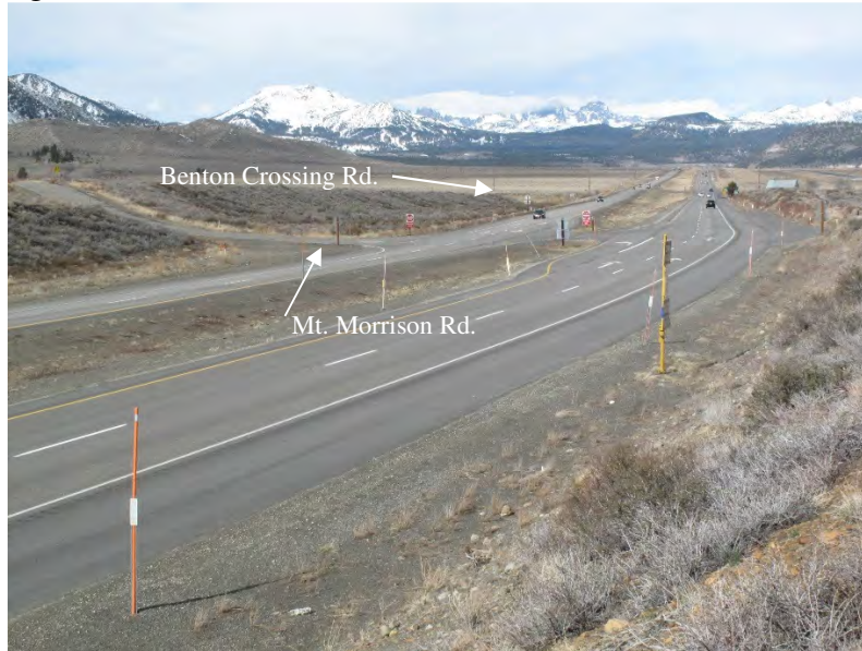
Image 2: US 395 looking to the north at hot spot no. 1 - the largest in the district.
