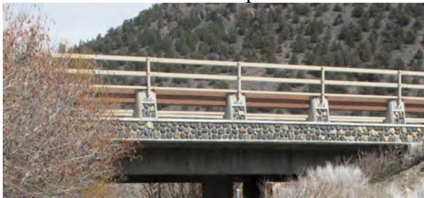
Image 5: Bridge railing and decorative features at Mammoth Creek bridges.
