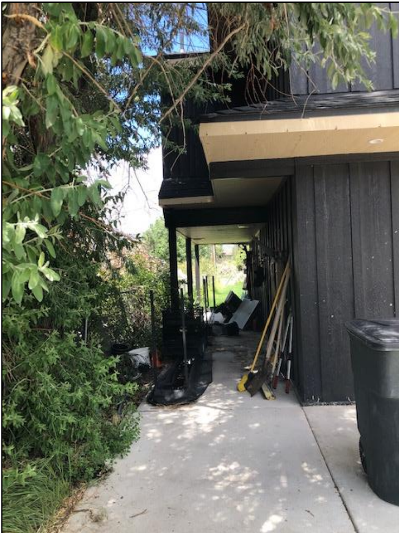
Figure 6. West side of residential unit.
