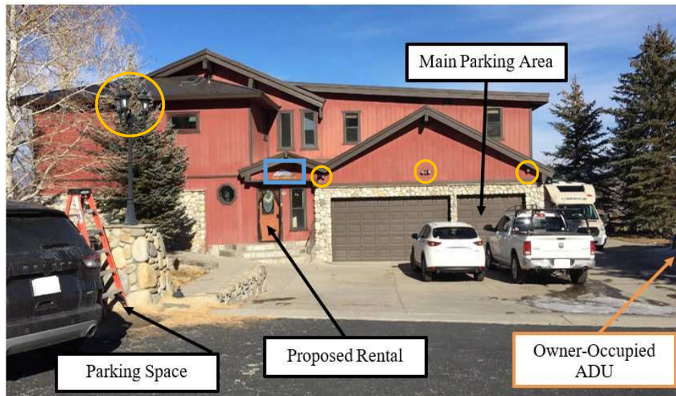
Existing exterior lighting and addressing on the proposed rental unit.
