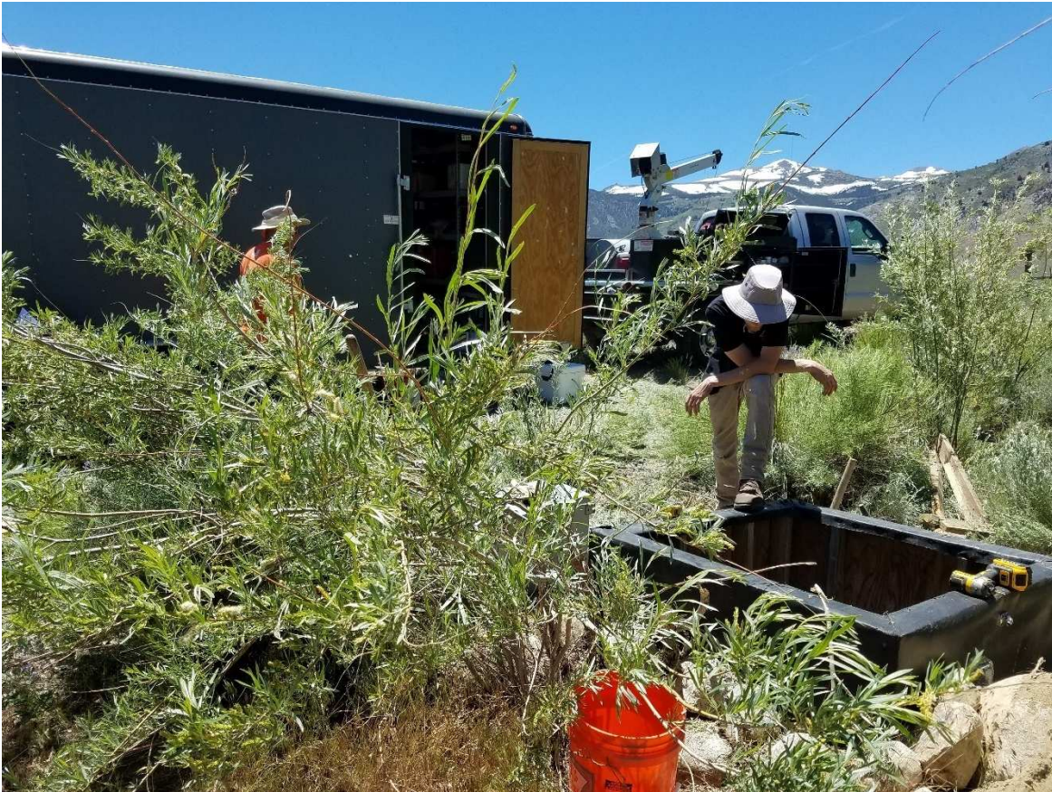
Sierra Geotechnical installing a flow meter and data logger on the Bowl Pipeline.
