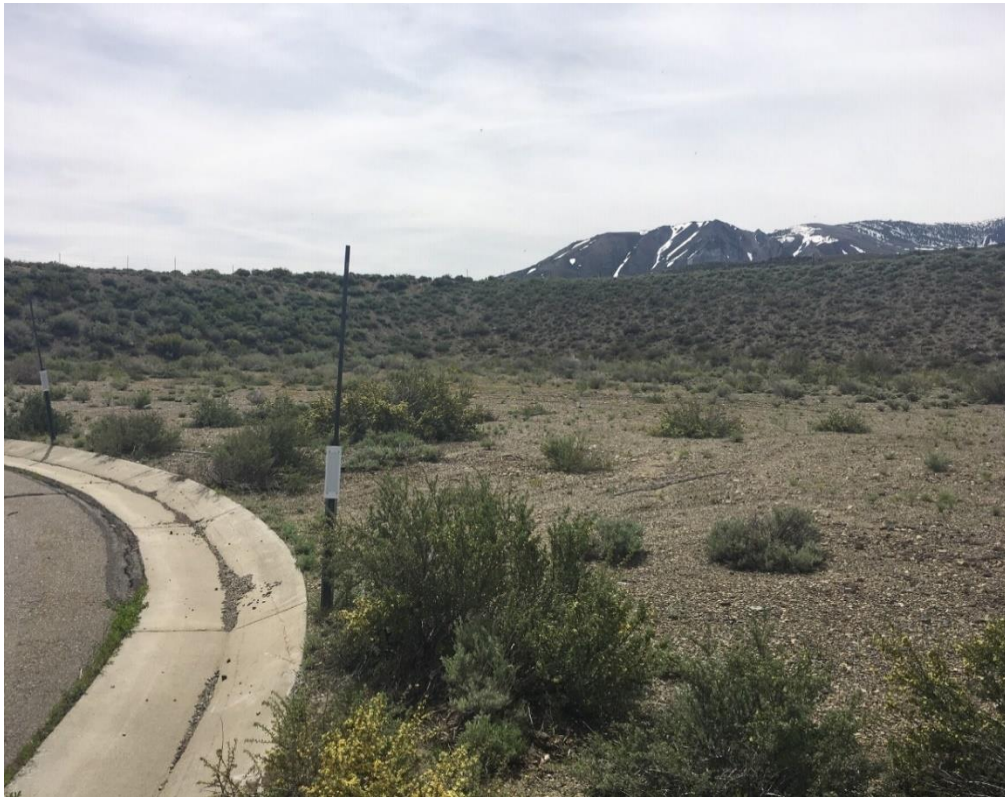
View of the project site and the Perimeter Maintenance Zone (PMZ) located on the south & east sides of the parcel.
