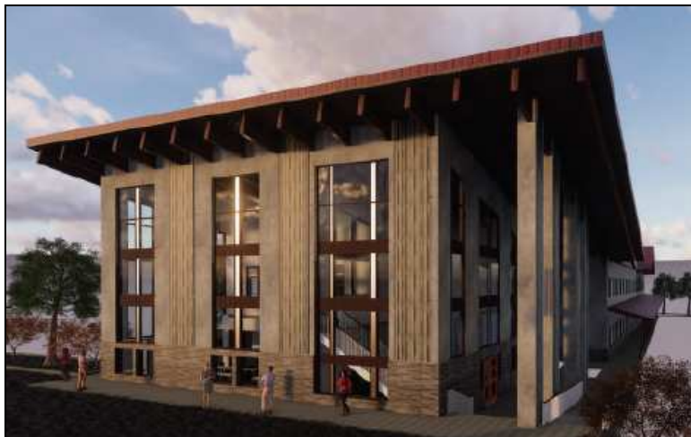
Plaza area, from the west
