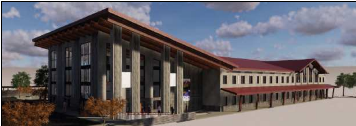
Main Entrance, from the southwest
