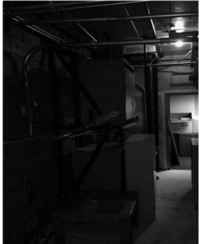
Electrical Image #4C – Washer Machine within Main Electrical Room
