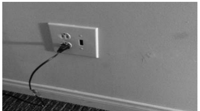
Electrical Image #12 – Duplex/Switch Type Coverplate
