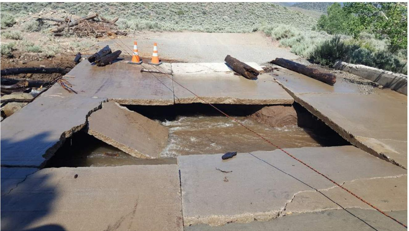
Photo 1 – Collapsed Concrete Slab Spillway – View West
