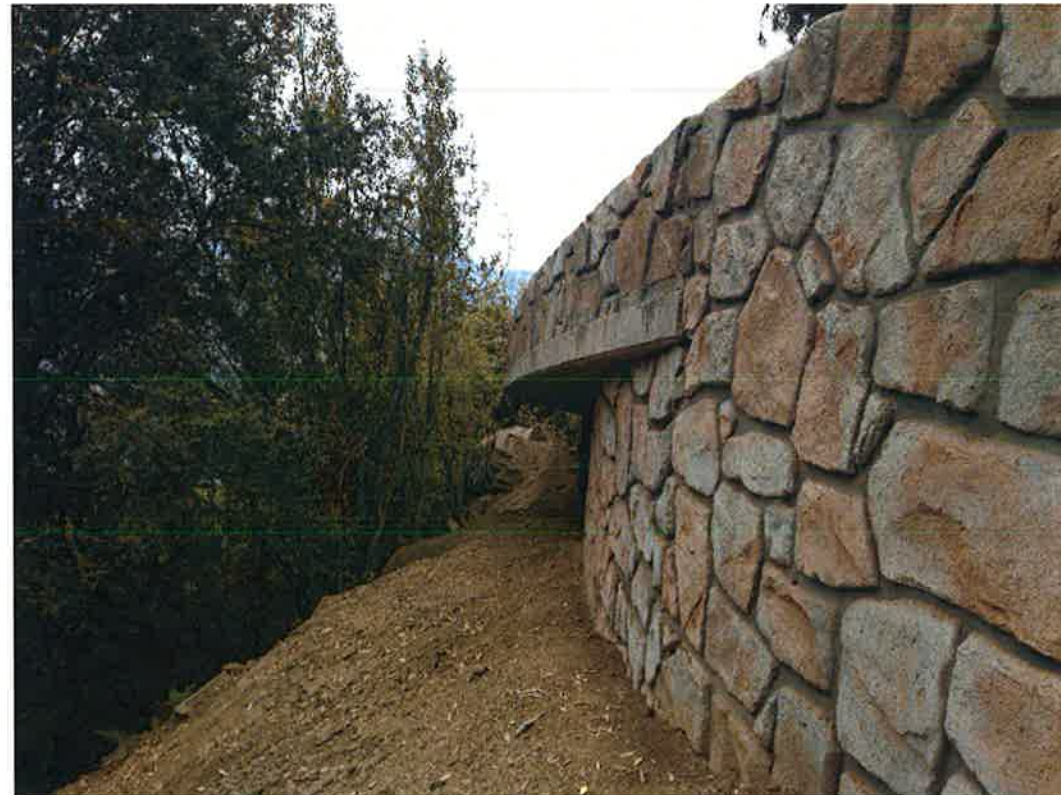
Photograph 7. Cast in Place Concrete Wall with Aesthetic Treatment
