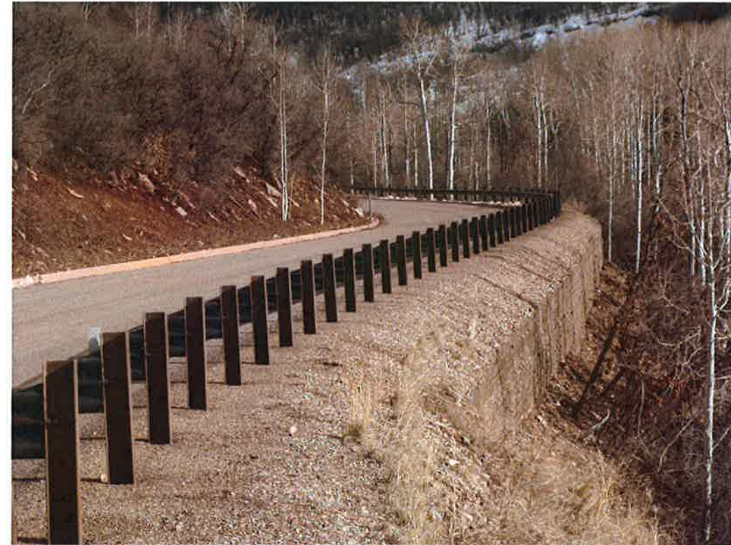
Photograph 2. Cast in Place Concrete Wall
