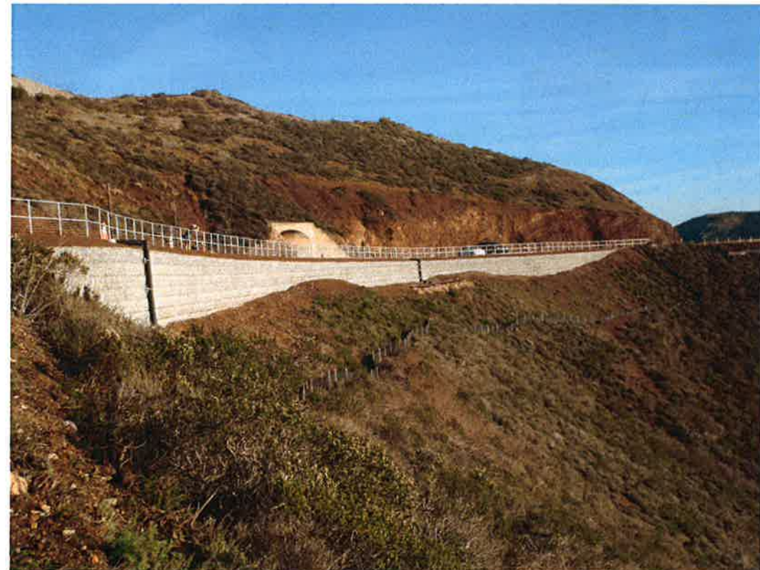
Photograph 4. Mechanically Stabilized Embankment Wall
