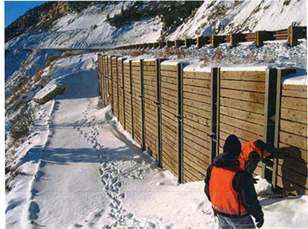
Photograph 6. Soldier Pile Wall with Timber Lagging
