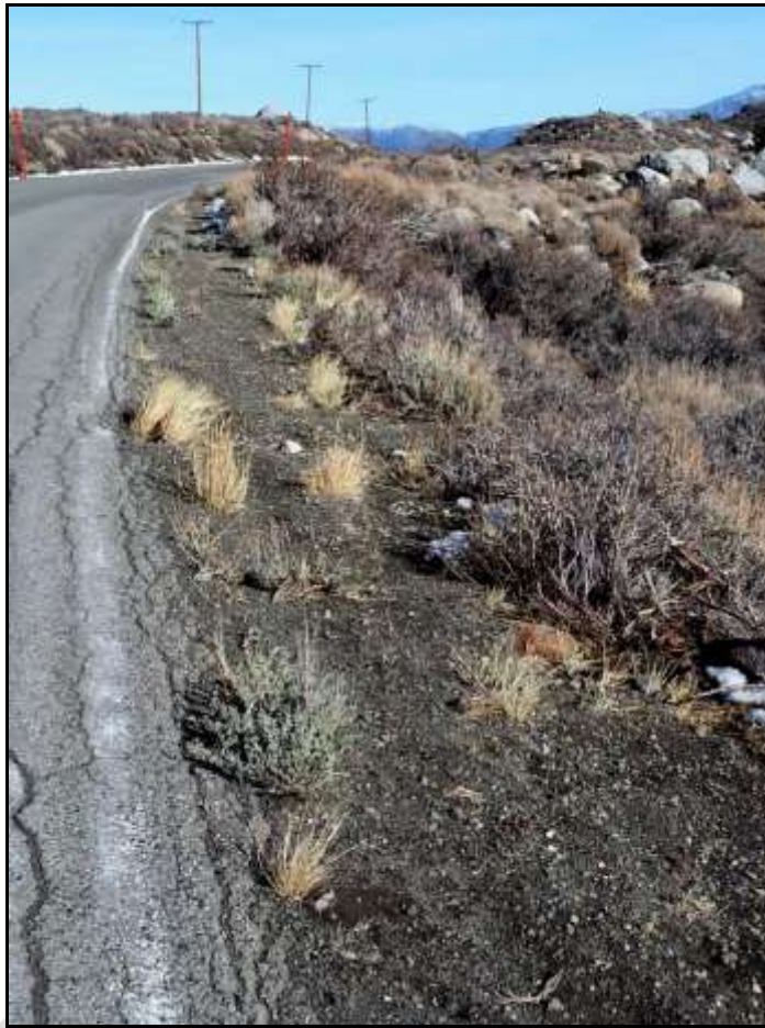
Figure 2. Typical roadside habitat that was searched on December 7, 2014 for Special Status plant and animal species presence. The major portion of Convict Lake Road passes through sagebrush scrub habitat, as shown here. An additional, smaller portion of the project will affect aspen riparian forest or willow riparian scrub.
