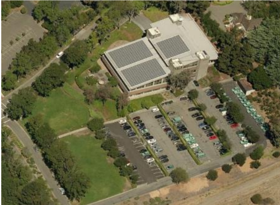
Figure 2.1: Overhead View of the District Headquarters
