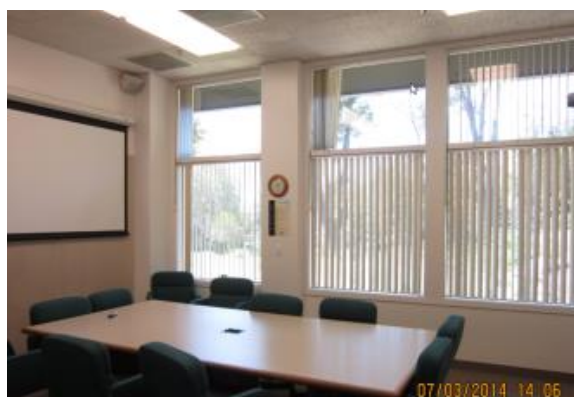
Figure 5.6: Lit, Unoccupied Room with No Manual Switch or Occupancy Sensor
