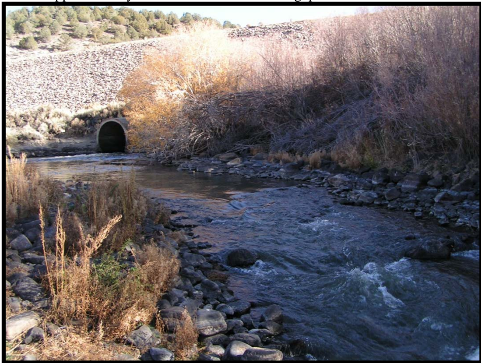
East Walker River looking upstream to Bridgeport Reservoir outlet.
