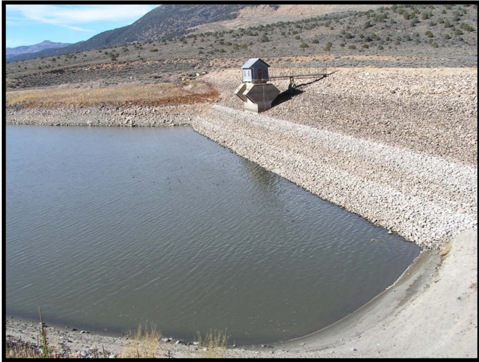
Bridgeport Reservoir dam and outlet control structure.
